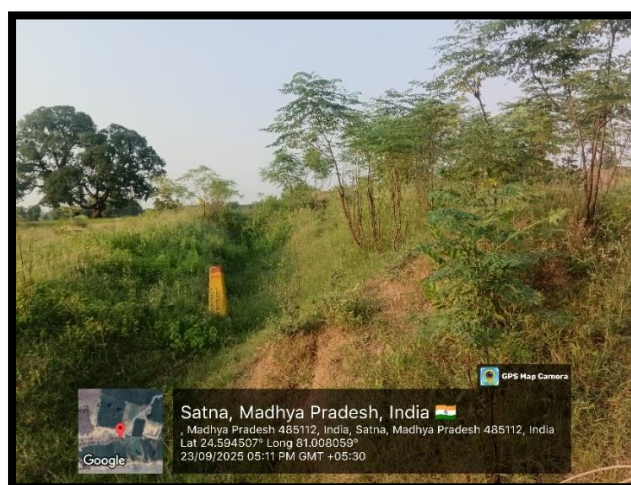
Garland Drain in Majhiyar Village
